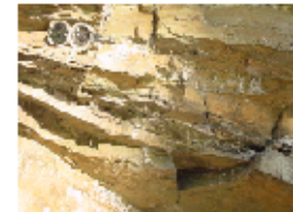
Fault Exposure In The Slab Sides Fm. Along Long Level (Black Ck.)
